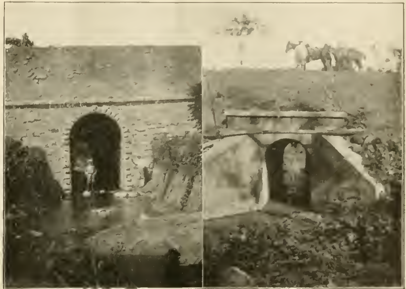
TWO CULVERTS ON THE EASTERN DIVISION, CUBAN RAILWAY.
